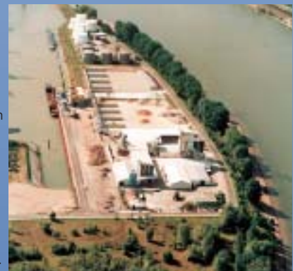
EC's contract processing plant Minera GmbH, on the Rhine at Andernach, Germany. Minera has a dry storage capacity of over 15,000m 2 . Courtesy Europe Commerce
